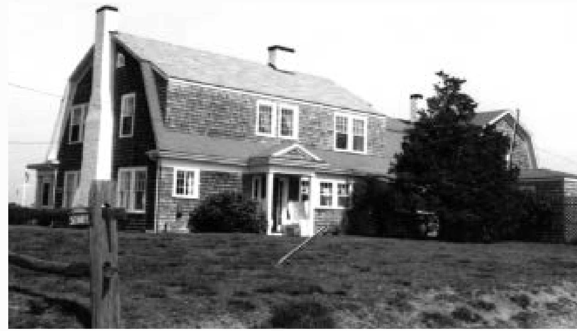
"Windyway" 9 Berkeley Ave 1920
